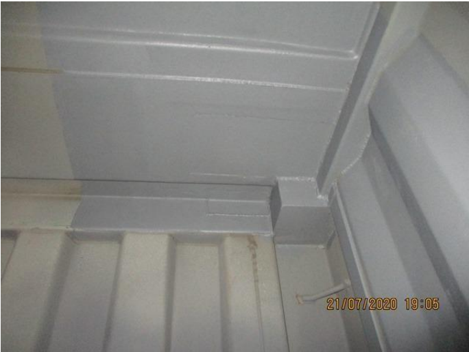
Proper replacement of the corner protection plate after installation of insert on the front header.
