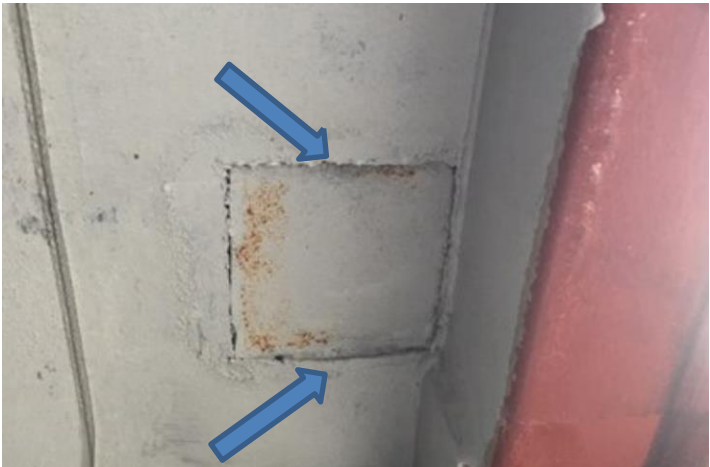
Non-conforming repair: insert installed on the corner protection plate however no insert installed on the extension plate.
