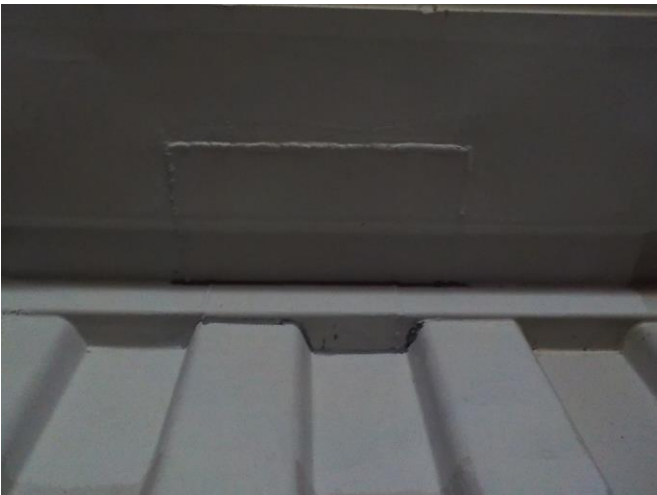
Proper insert to the header extension plate.
