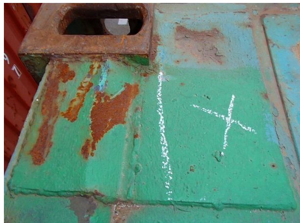
Acceptable insert on corner protection plate. Any damage to the header must have been repaired prior to insert installation.
